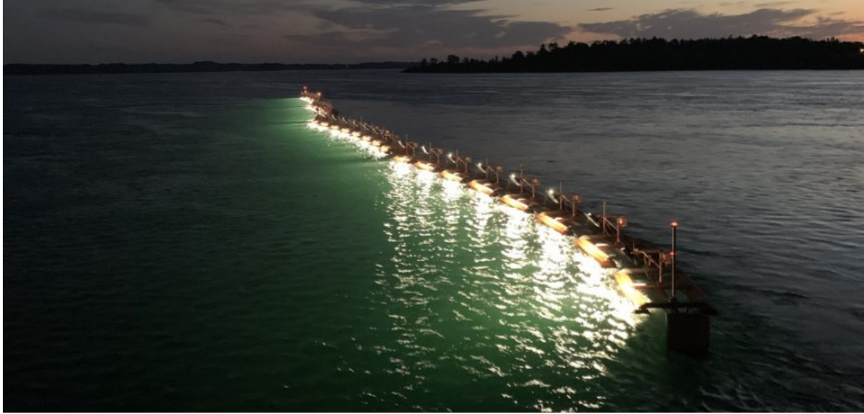
Figure 3. Photo of the 216 m long experimental light guidance array deployed upriver of the Iroquois Water Control Dam with the goal of behaviourally guiding out-migrating American Eel Anguilla rostrata to collection and safe passage, Fall 2022.
